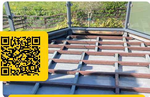
BATTENS, JOISTS & SUPPORT PEDESTALS
